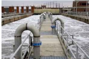
AP – In this photo taken on Feb. 26, 2009, aeration basins are seen in operation at the Wilmington Wastewater ...
