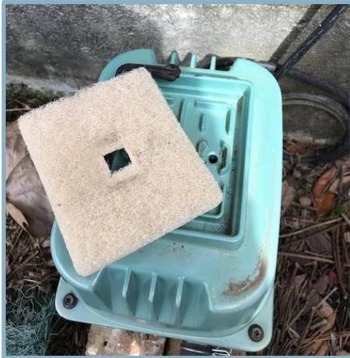
*Figure 1: Well-maintained, properly functioning home waste system aerator*
