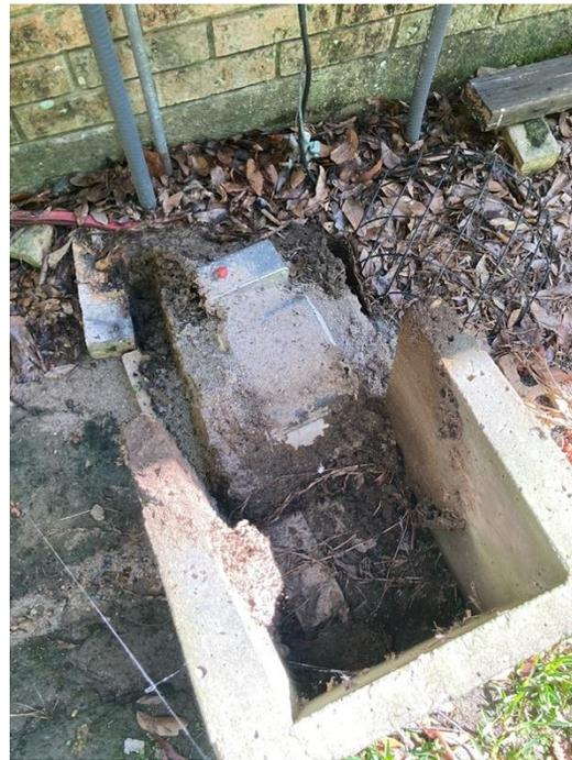
Figure 2 – Aerator covered in ants and not working
