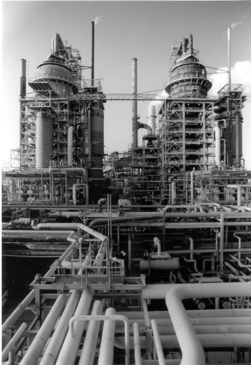
Catalytic cracking technology invented at Exxon Baton Rouge in 1942 helped win WWII. It remains industry standard.
