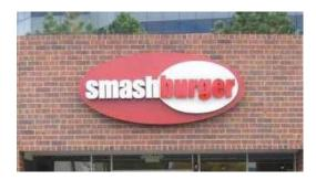
One final backer panel design consideration - reverse lit channel letters should not be mounted to a glossy backing panel surface. Doing so generates a sort of "mirror image" on the panel and the actual LED modules (and sign wiring) may be seen in the sign reflection. Obviously, this is undesirable. It is much better to use a matte or satin finish when mounting reverse lit letters to a backer panel.
