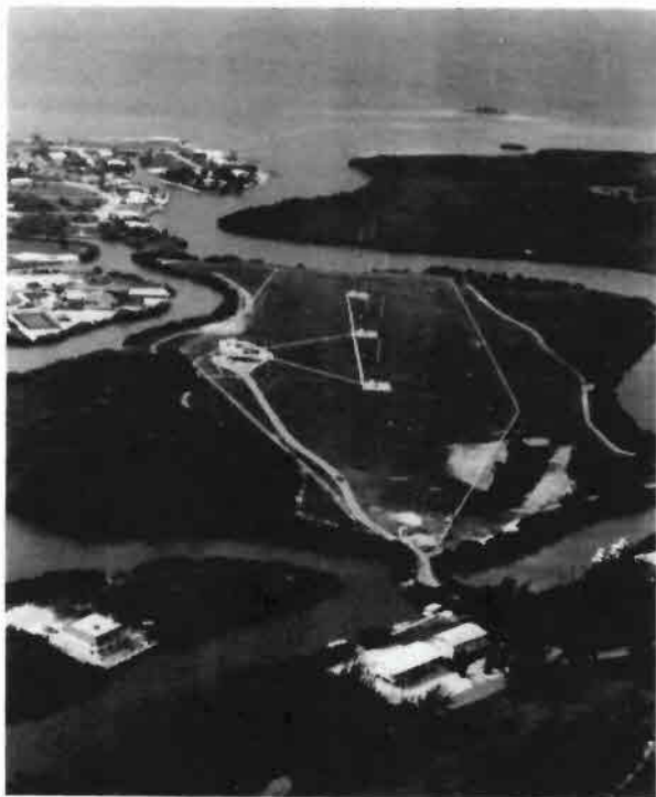
VOA's Radio Marti program is fed by satellite from Washington to this relay station in Marathon Key, Florida for broadcast to Cuba on a 50 KW medium wave transmitter.
